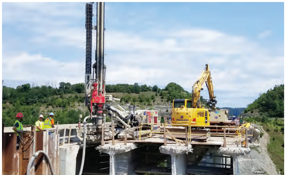
CJ Mahan at bridge job in Mason County
