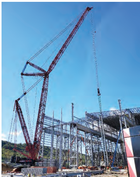
Mammoet Crane at Nucor Steel in Gallatin County, Kentucky
