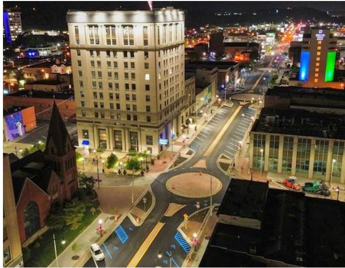
View of The Newly Installed Roundabout in Ashland KY Allard Excavation
