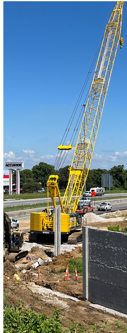
Ragle, Inc. setting sound walls on the I69 project
