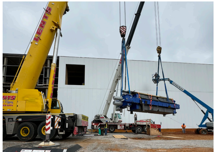
Lents Crane & Rigging at Ascend Battery Plant in Christian County, KY
