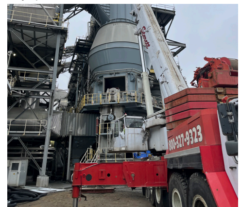
Sterett Crane & Rigging at Heidelberg Materials in Mitchell IN
