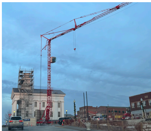
R. H. Marlin At Paoli, IN, Repairing Clock Tower
