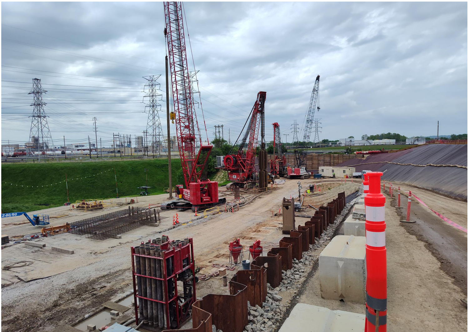
Nicholson Construction at Paddy's Run
