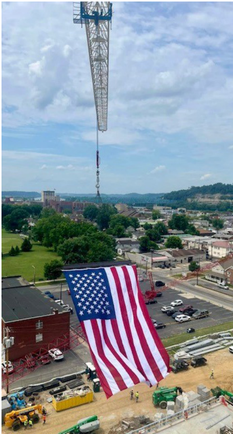
DS6 Daryl Wells Tower Crane view at KDMC Ashland, KY
