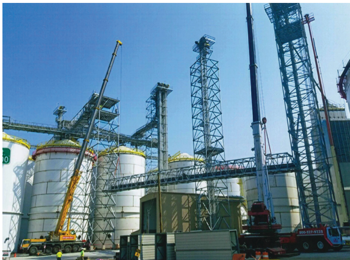
Barnhart Crane & Sterett Crane making a double pick at Owensboro Grain in Daviess County, KY
