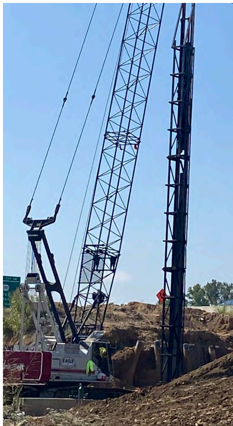
DS1 Eddie Bennett driving piling on I-69 for Ragle Inc. in Henderson, KY.
