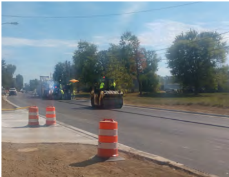
DS 3 Paving project for Milestone Contractors.
