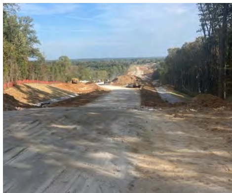
DS 3 Lutgring Bros. Inc. State Road 64 project in Waynesville, Indiana.
