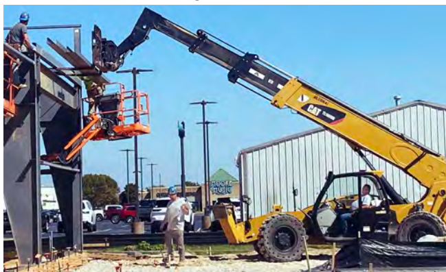
Scott Goelzhauser with Enerfab at Expressway Dodge in Evansville.
