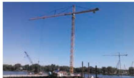
Walsh-Vinci working on Section 5 of the East End Bridge
