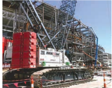
Maxim Crane setting iron on UK Commonwealth Football Stadium in Lexington, Kentucky
