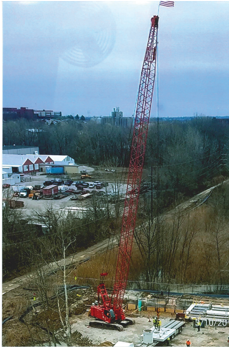
Kokosing on the Westside Treatment Plant expansion in Evansville, IN
