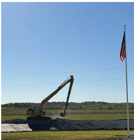
DS 1 Barnard Construction at TVA.
