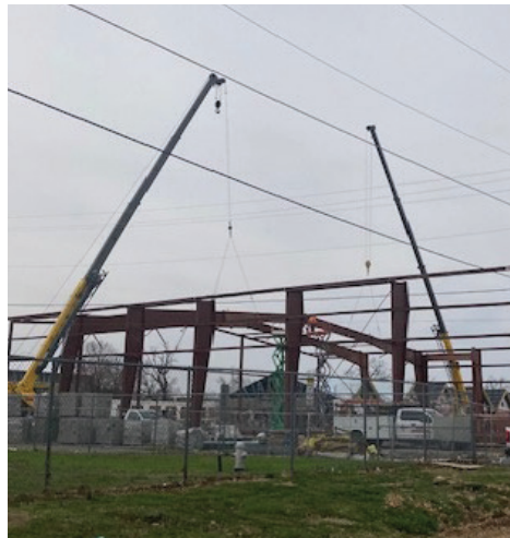
DS 5 Marshall Crane setting iron on Paducah Head Start.
