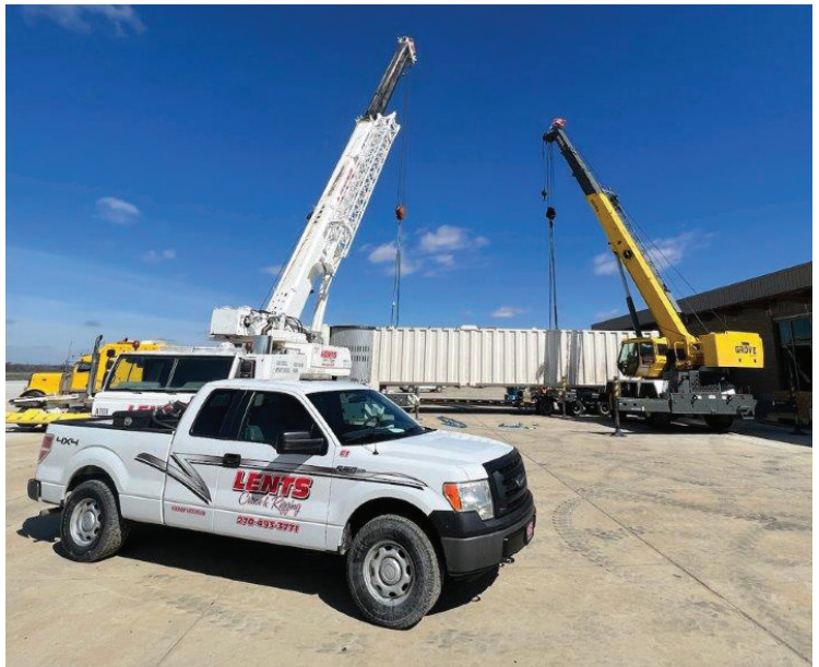
Lenis Crane working at the Barkley Regional Airport.
