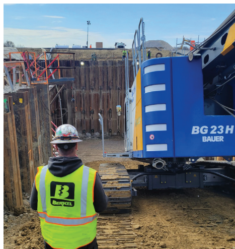
DS 2 Berkel & Company and Bowen Engineering at Wansford Yard Lift Station.
