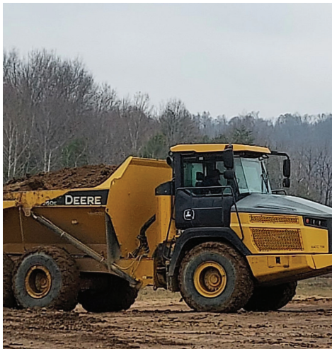
JATC-Boston Ricky Jones operating the Articulating Truck while hauling fill for projects
