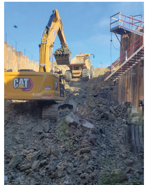
Bowen Engineering at Wansford Yard Lift Station.
