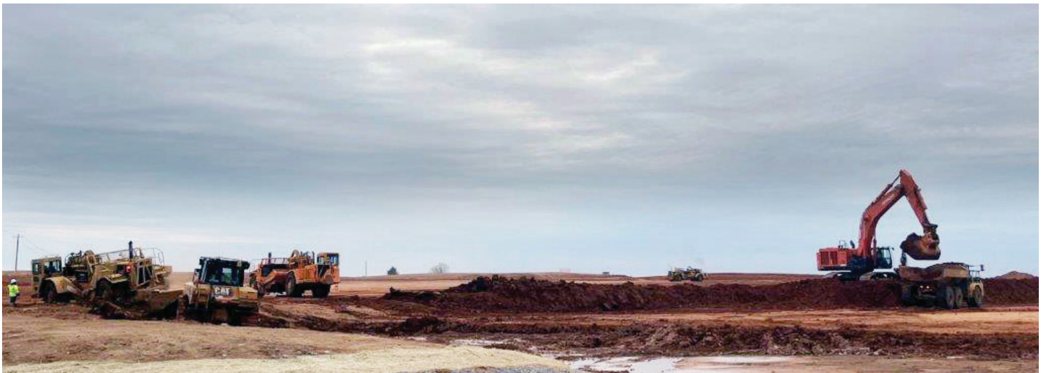
Kokosing Industrial working at the Ascend Battery Plant in Hopkinsville, Ky.
