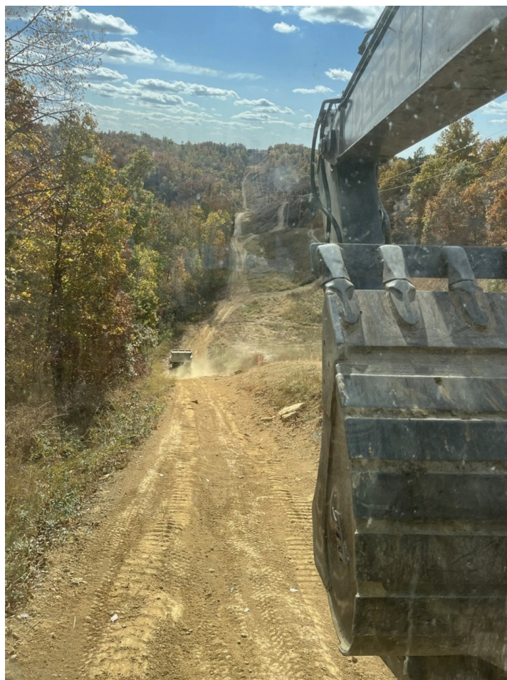
Contractors Rental working in Cannonsburg, Ky.
