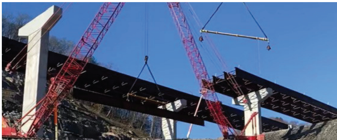
Setting beams in Elkhorn City, Ky.
