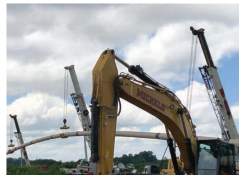
Michels Pipeline in Mercer County, Kentucky
