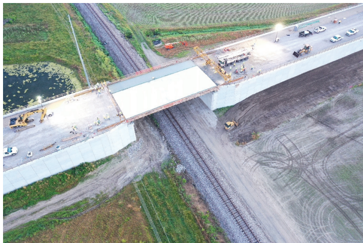
Milestone Bridge work
