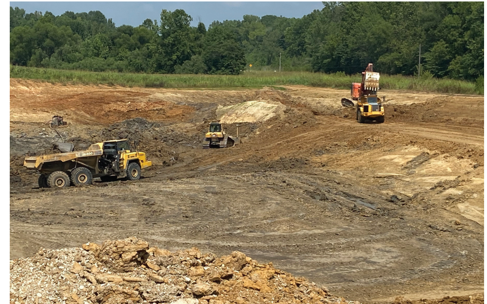
Blankenberger Bros at IPL power plant ash pond Closure
