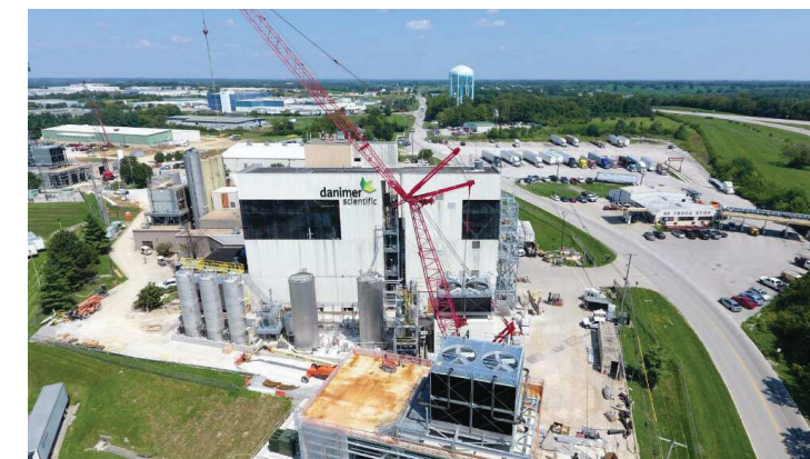
Lattice Boom Crawler being run by Charles Rogers at Winchester dairy
