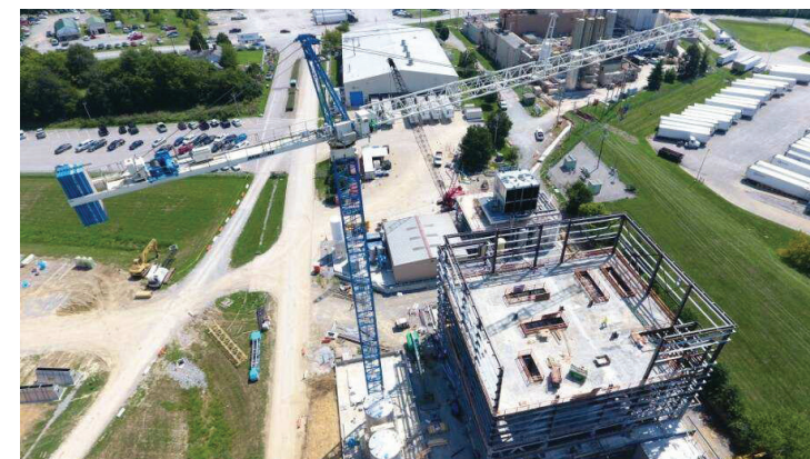
Tower crane being run by Frank Miller at Winchester dairy.
