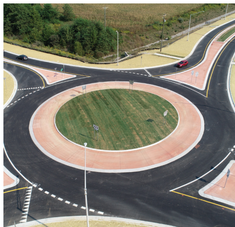
E & B Paving Salem Roundabout
