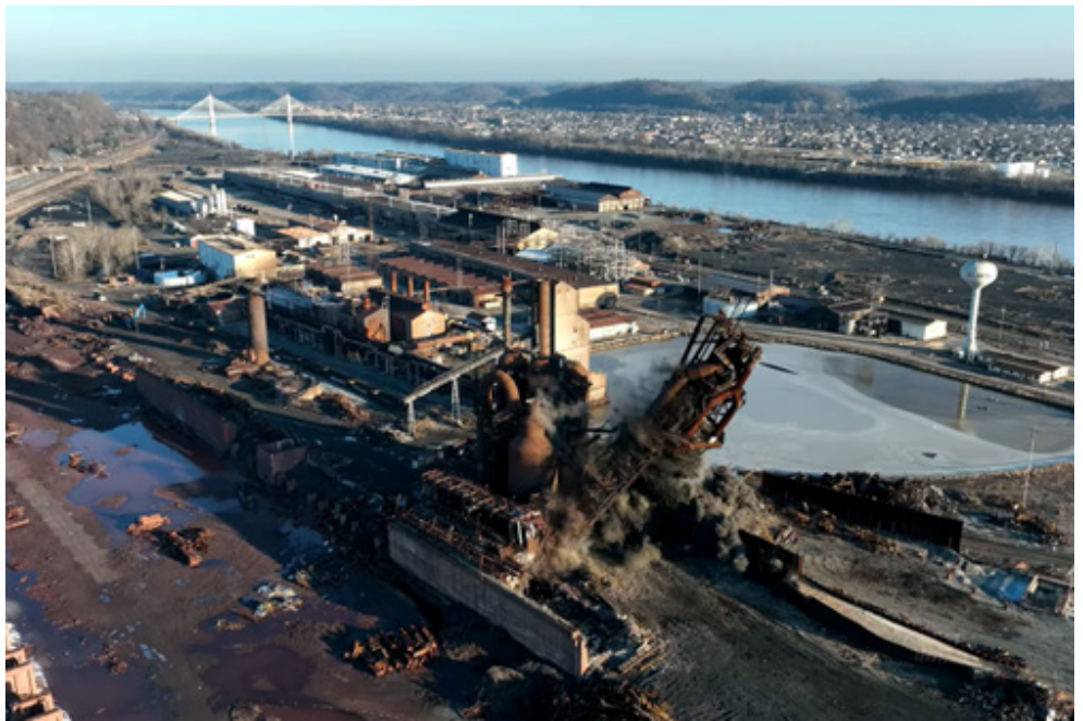
AK Steel Demolition
